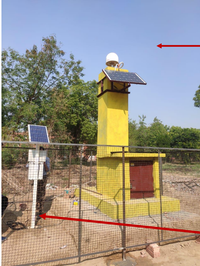
Ex. GNSS and Soil Moisture Probes Installed at JNV, Sirsa, Haryana.
